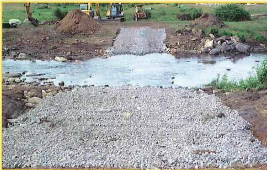
Figure 6. Construction and final grading of upstream cattle crossing.
