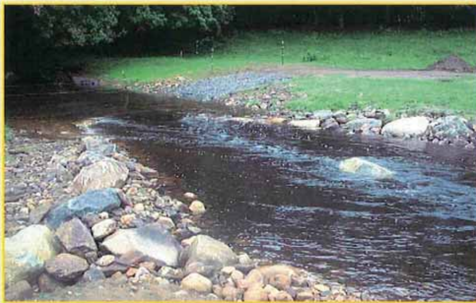
Figure 2. Photograph of cross vane 12+10 during a storm event illustrating a primary function of the cross vane to redirect flow into the stream's centerline and away from the streambank.
