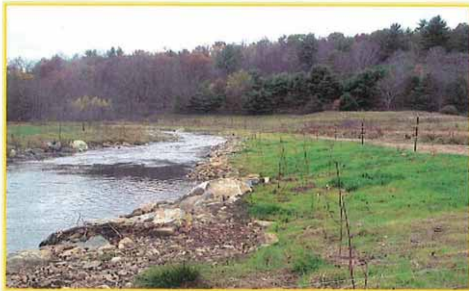
Figure 10. Photograph showing vegetation reestablishment along bankfull bench.
