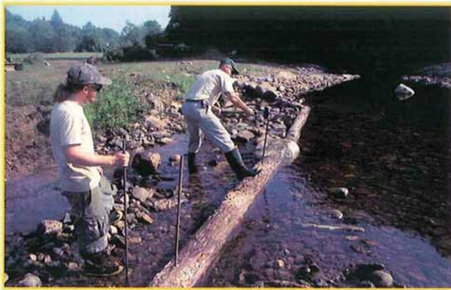
Figure 5. WHAMM staff installing reinforced bar to secure bank placed logs.
