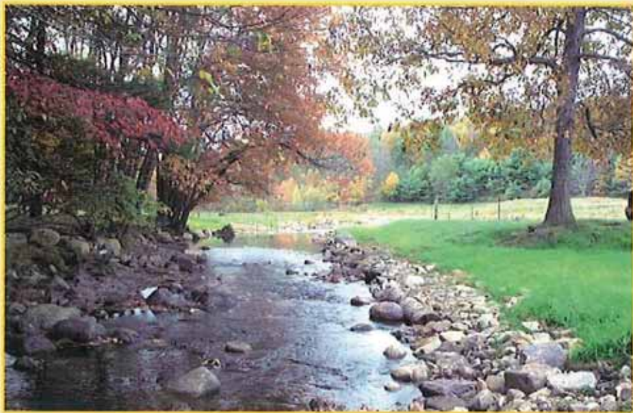
Figure 12. Post construction photograph of narrow channel and creation of bankfull bench.
